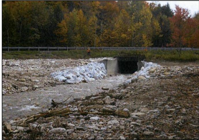
**Figure 3.1:** Repairs to washed out wingwall abutment and retaining wall at the outlet of a Route 7 culvert near the Glastenbury-Shaftsbury town line.
