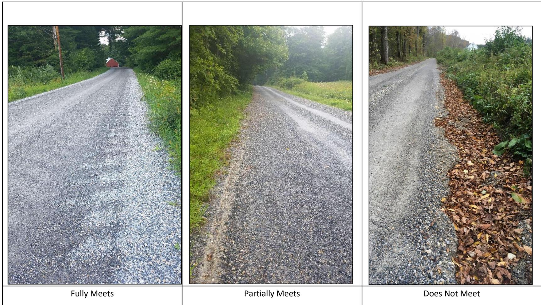
**Figure 4.3:** Examples of road segments with different levels of MRGP compliance.
